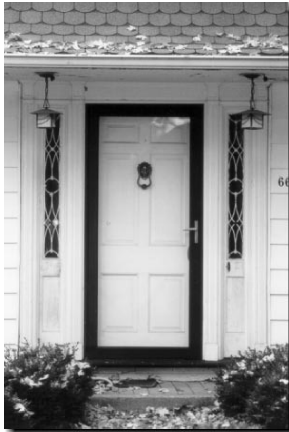
{PHOTO 55} A full light metal storm door will show as much of the door as possible.
