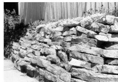
{ PHOTO 83 } Dry laid split rock retaining wall.
