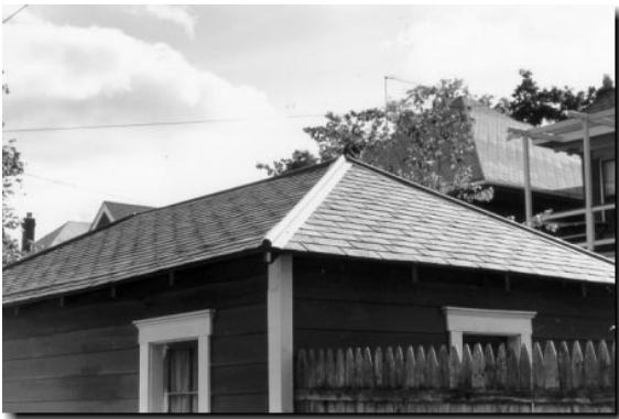
{ PHOTO 24 } Asphalt shingle with a metal ridge cap.
