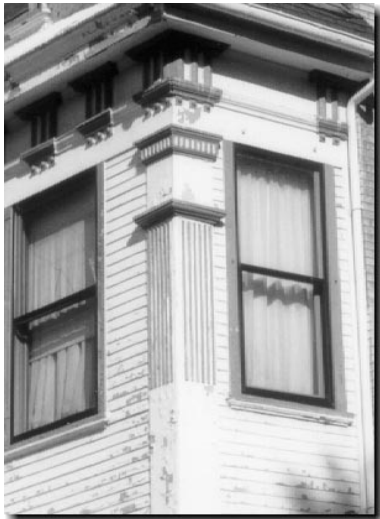
{ PHOTO 37 } Storm window with a meeting bar in the same place as the window's meeting bar.
