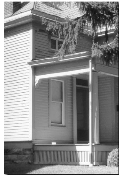
{ PHOTO 7 } Many wood structures have corner boards with wide trim around windows and doors to match.
