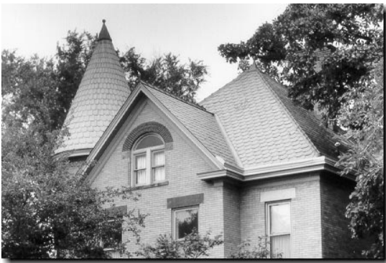
{ PHOTO 22 } Slate roof with ornamental metal ridge roll.
