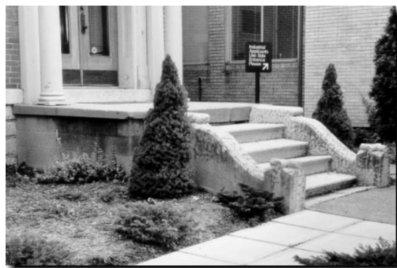
{ PHOTO 5 } Limestone steps, common for this district, lead to a small stoop. Note a small post sign to the right of the stoop which helps to direct some pedestrian traffic.
