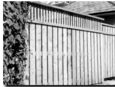
{ PHOTO 70 } This board-on-board six-foot privacy fence has a top fence detail that helps break up the horizontal plane. Also, the "dressed" side of the fence is facing out and the framing is toward the inside.
