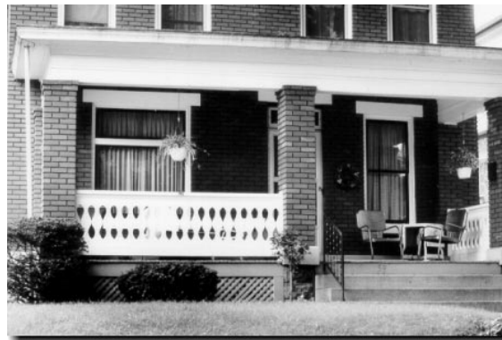
{ PHOTO 4 } An example of a decorative panel, one of many different types of porch screening.
