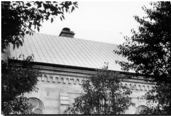
{ PHOTO 23 } Standing seam metal.
