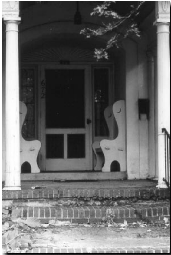
{PHOTO 54} This wooden storm door repeats the pattern of the door.
