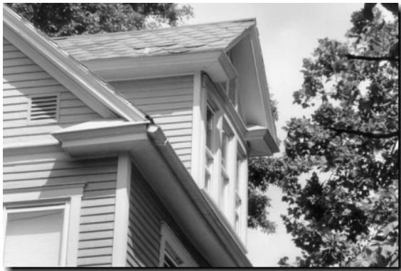
{PHOTO 31} Wood-sided dormer with corner boards to match the rest of the house.
