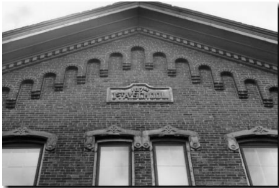
{PHOTO 13} An arched masonry cornice detail with a wood overhang.
