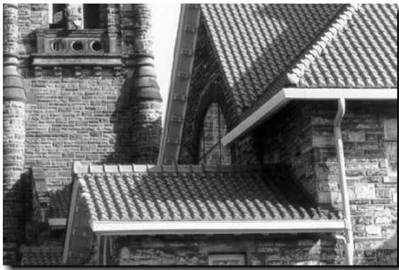
{ PHOTO 21 } Red tile roof with tile ridge cap.
