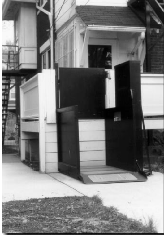
{ PHOTO 78 } Even in tight spaces accessibility can be achieved with a chair lift.
