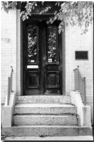
{ PHOTO 3 } Stone steps and stoop with a simple metal handrail.
